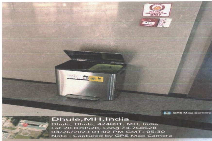
Solid and Bio Waste collection dustbin available at every floor of institute building
